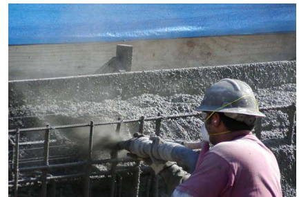
Concrete with KF-A applied by shotcrete without plasticizer & water reducer.
