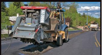
"We're able to grind a 1000 feet long ditch 9
