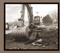
Generally, the old asphalt has to be ripped up and hauled off, the subsurface replaced with new fill, the roadbed recompacted, and the road repaved.
